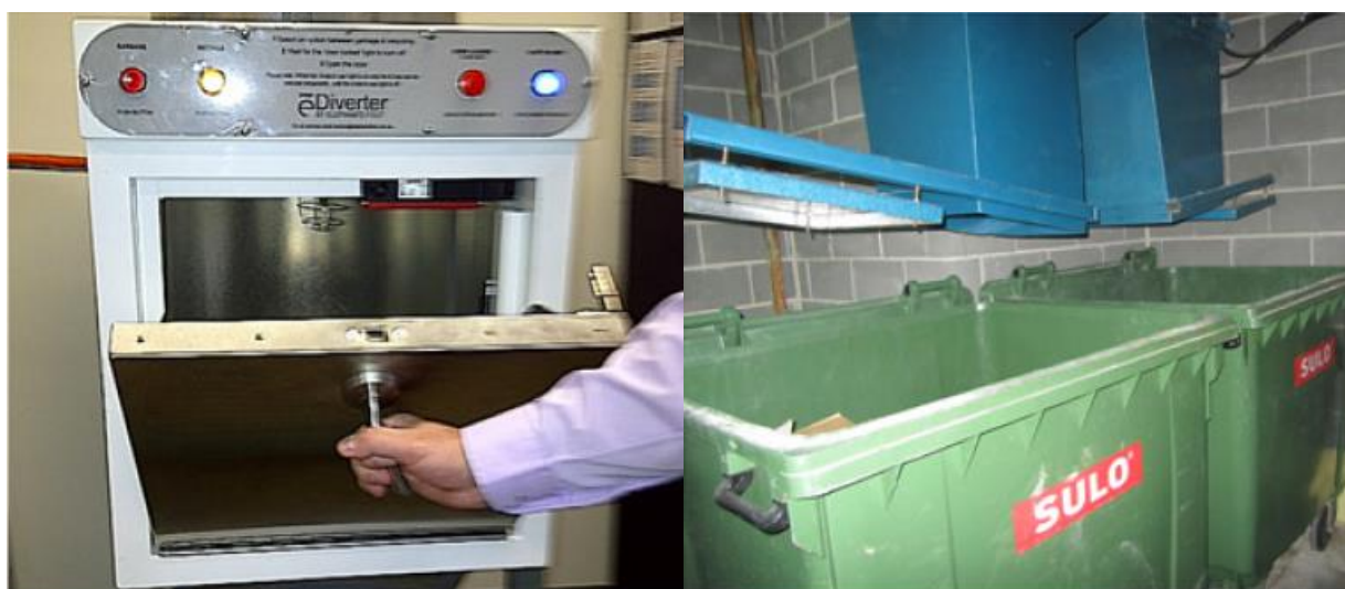
Figure 1 eDiverter Waste Chutes for Residential Multi-use Developments
